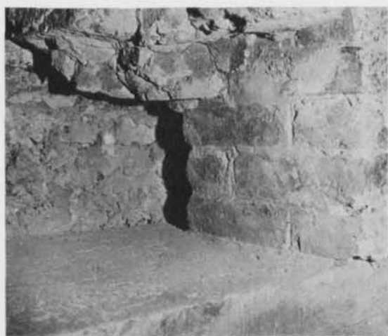
Bild 2. Bild från framtagningen. T. h. de fem bevarade skiften av smygen i den port, vari Medusastenen lagts som tröskel. Observera tegelmurverkets planstrukna fogar med bred rits. Foto M. Svendsen 1971. — Picture showing a stage of the exposure. To the right, five courses of the doorway in which the stone served as threshold. Observe the joints, flat-rubbed with broad scratches.
